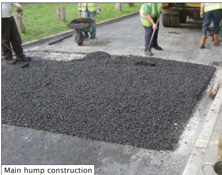
Inner section of the hump being laid
