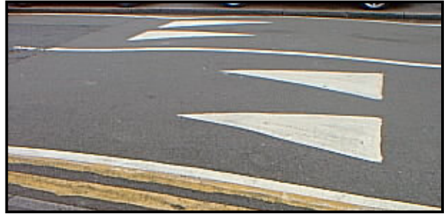
Proposed sinusoidal road hump
